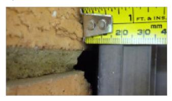
**Figure 9** A gap on the external wall surface between frame and brickwork.
