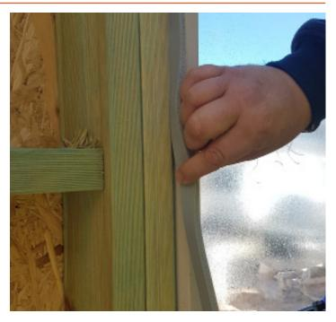
Figure 11 Applying high density acoustic foam
